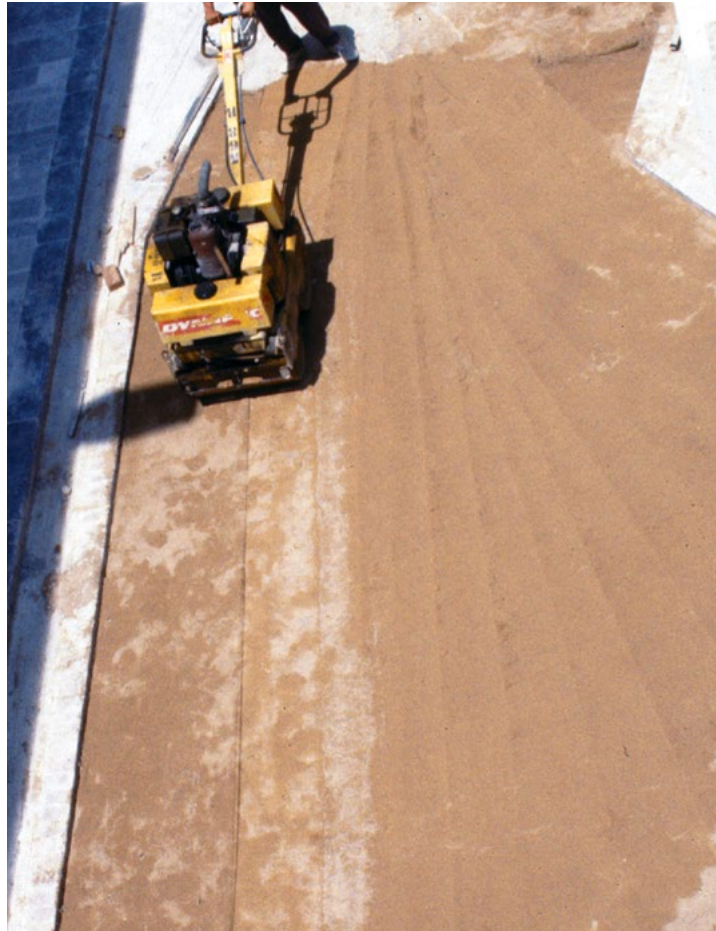
Levelling and sand compaction
